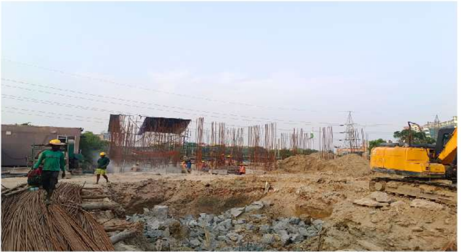
TOWER-1, PILE BREAKING WORK IN PROGRESS
