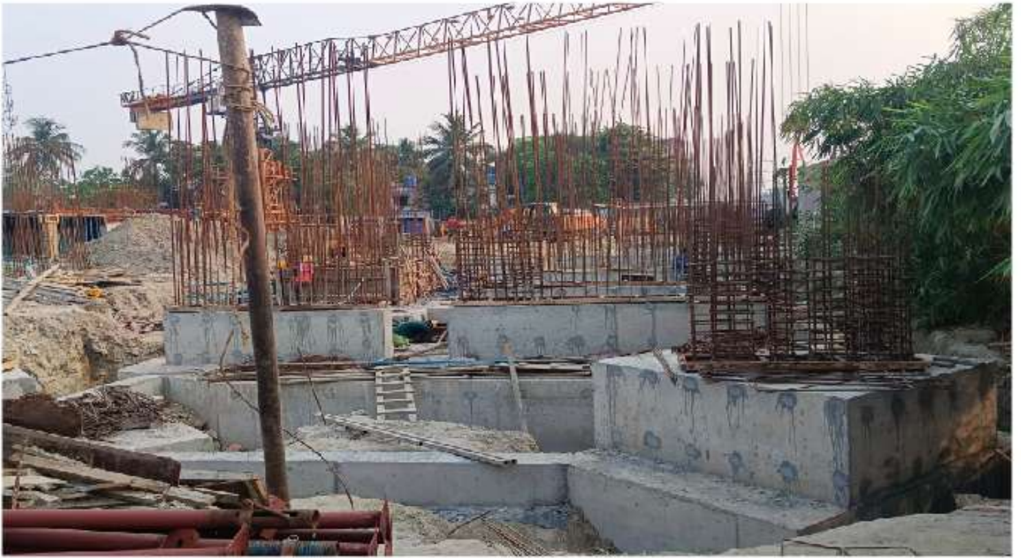
TOWER-1, PLINTH LEVEL REINFORCEMENT WORK IN PROGRESS
