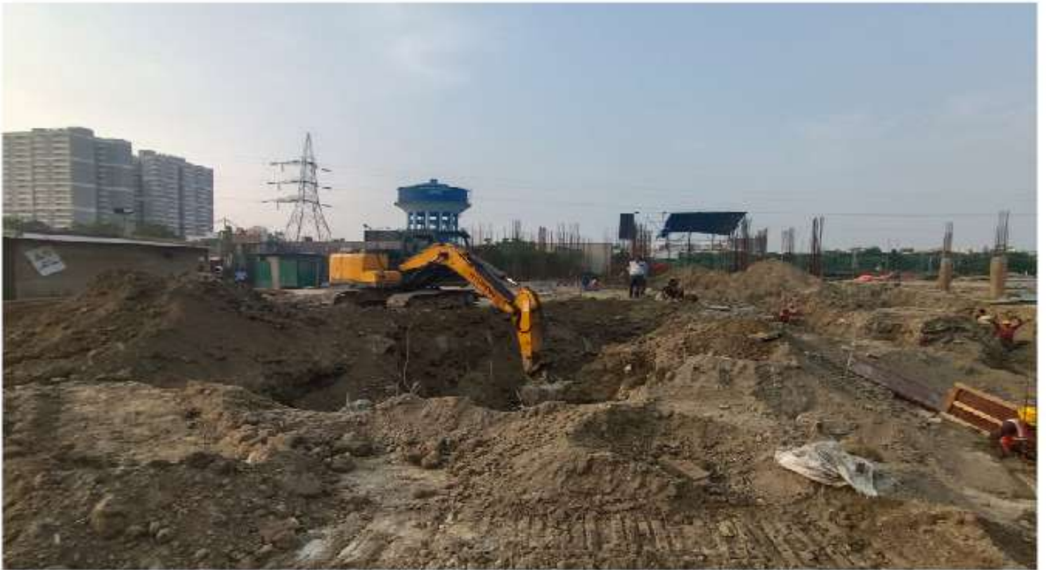
TOWER -1, PILE CAP EARTHCUTTING WORK IN PROGRESS
